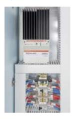
3. Verify all field wiring according to drawing package and turn all breakers to the <u>OFF</u> position.
